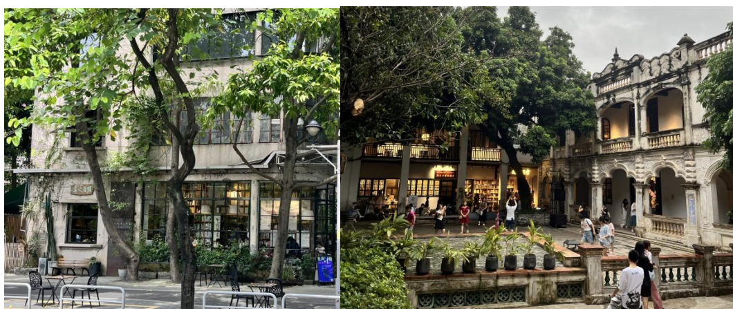
Figure 1: The view of the Sensing Bookstore and a part of the Lingnan Tiandi (Longtang Poetry Society).
