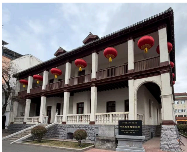
Figure 1. Hedong Salt Administration Audit Sub-bureau
